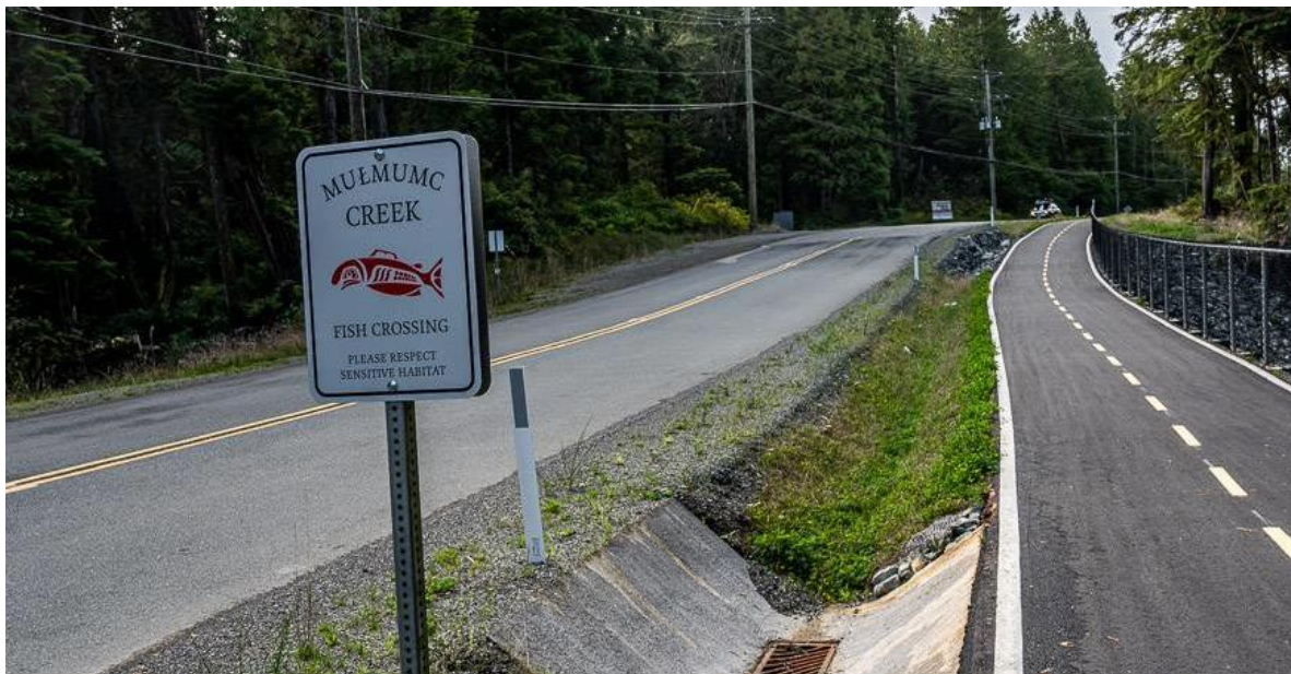
The new multi-use pathway in Tofino is an example of an active transportation facility that meets the ultimate standards. With signage, asphalt, pavement markings, and drainage ditches, this 25 kilometre multi-use pathway will make it much easier for people to walk, roll, and cycle within and around Tofino. Photo credit: Hike, Bike, Travel.
