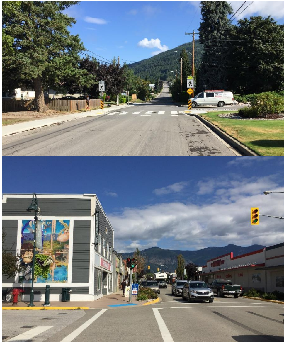
Examples of crossings in the Town with a raised crosswalk (top) on 20 Avenue South and a standard crosswalk (bottom) on 11 Avenue North and Canyon Street.
