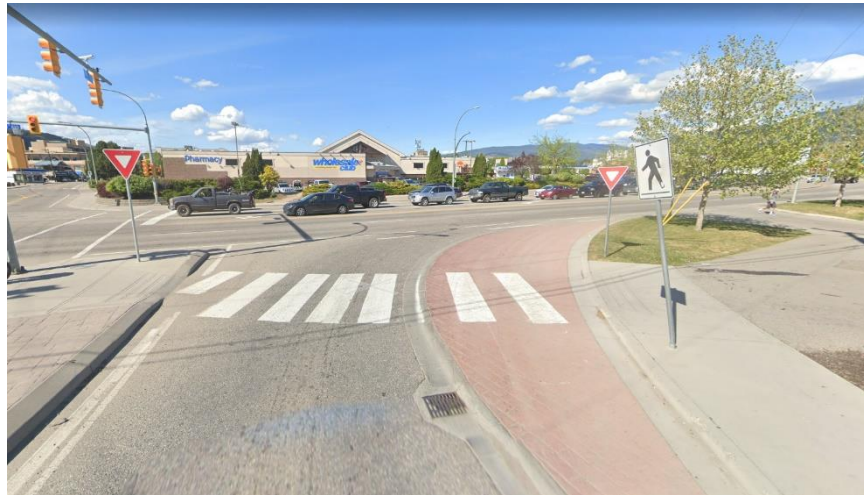
Truck apron in Vernon, BC at the intersection of two highways.
