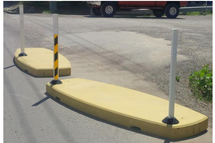
Temporary Traffic Curbs
