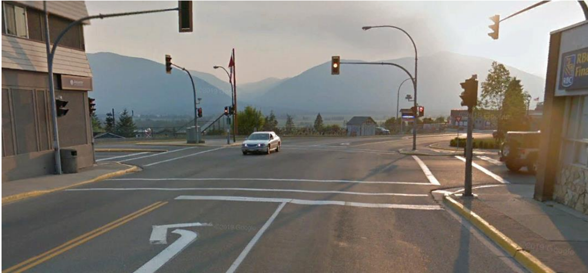
Cook Street / Canyon Street (Hwy 3) / 10 Avenue N intersection looking west. Building on left side of photo creates a sightline concern for northbound traffic and the pedestrian crossing on the east leg.
