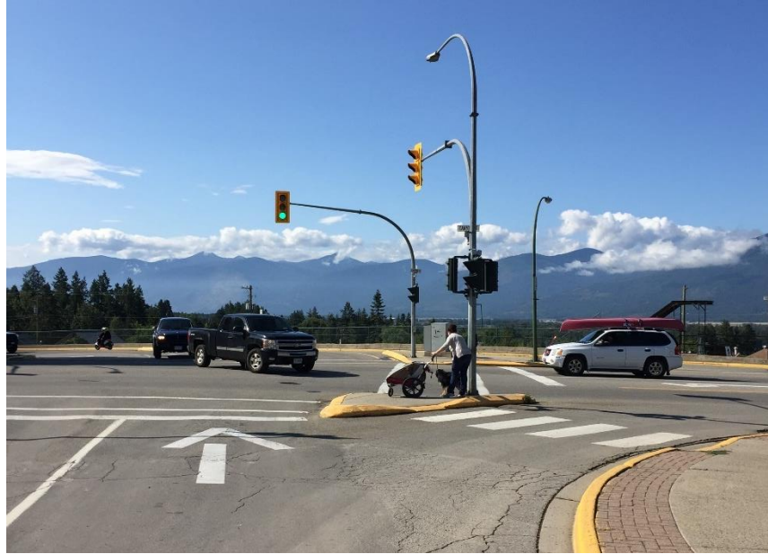
Channelized island on NW corner of the Cook Street / Canyon Street (Hwy 3) / 10 Ave N intersection can only fit person/bike/stroller
