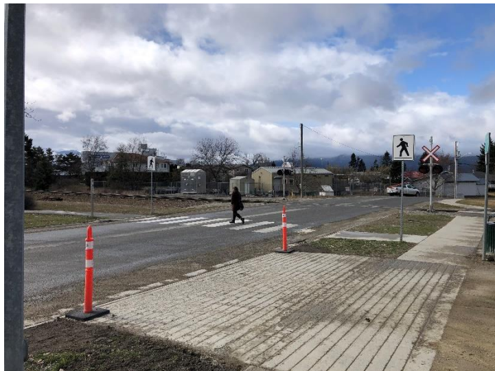
Example of a separated sidewalk on Cedar Street west of 16 th Ave S
