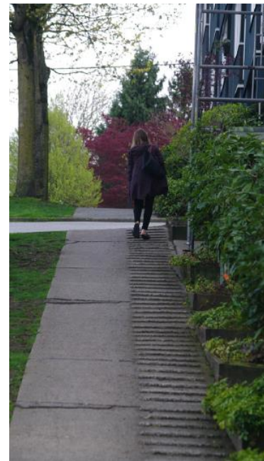
Example of a ladder sidewalk. Retrieved From: BC Active Transportation Design Guide
