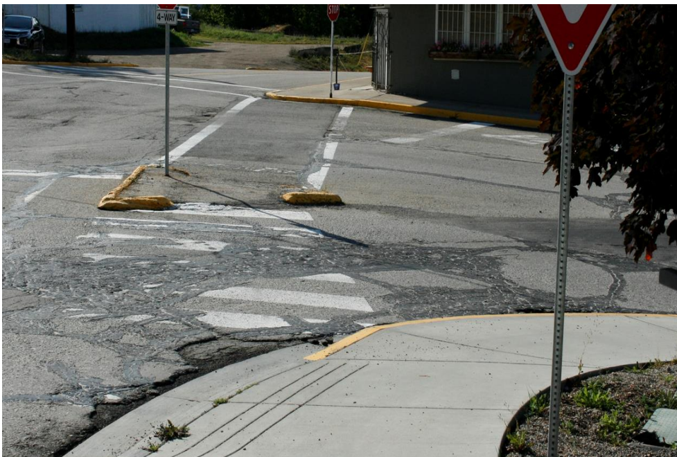
Example of curb ramp in the Town that has been modified (foreground), an unmodified curb ramp on the channelized island and a vertical curb with no ramp on the far side of the intersection located at 9 Avenue and Canyon Street
