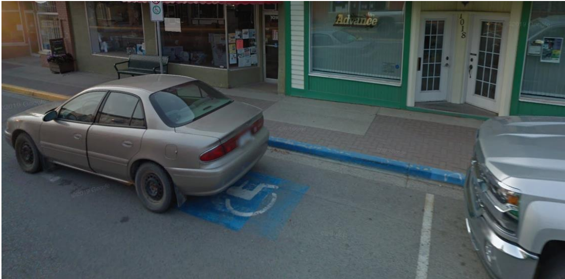
Example of an accessible parking space on Canyon Street. While the space is well marked with signage, a blue painted curb, and a pavement marking, there is no curb ramp and there is limited space for those using a rear lift to enter/exit their vehicle.
